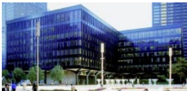
Building 4 of the World Trade Center
