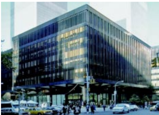
Building 5 of the World Trade Center
