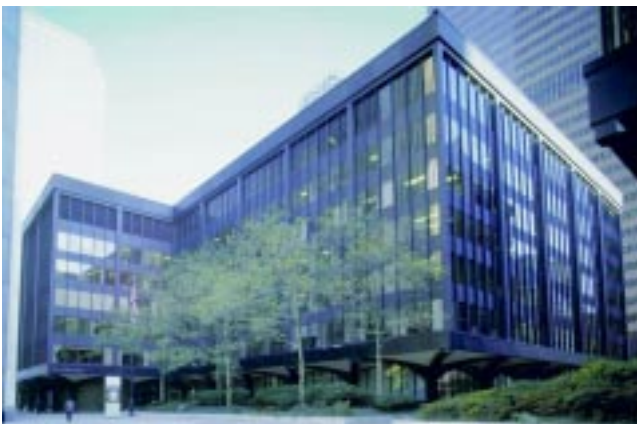
Building 6 of the World Trade Center
